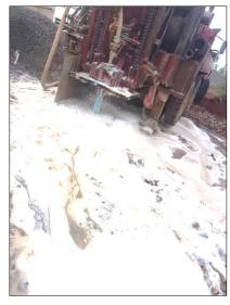
The water well crew is busy drilling 20 additional wells in the Sidama Region of Ethiopia. They sent these pictures in mid-June as they were drilling well #5 of the 20. We didn't know what the white foam was and they reported it was used to coat the walls of the borehole to keep it from collapsing! They are enjoying the great ministry of providing pure clean water for the people of Sidama.
